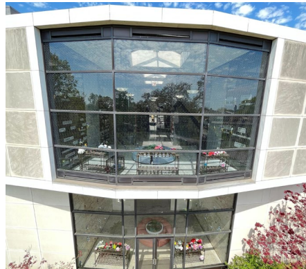
Green-Wood Cemetery's Hillside Mausoleum now has almost 20,000 sq. ft. of bird-safe glass.
