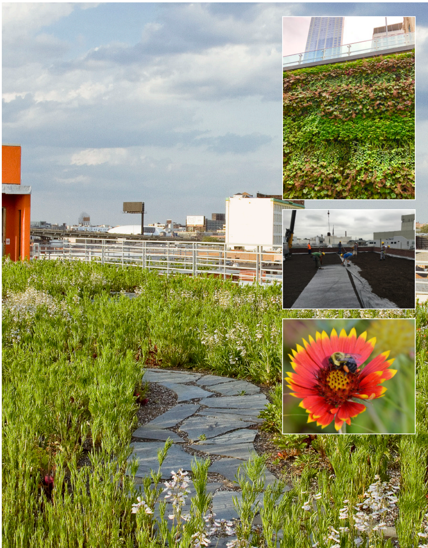
Intensive green roof at Kingsland Wildflowers at Broadway Stages. Insets from top: Living wall at the 9/11 Memorial & Museum. Installing soil medium at Kingsland Wildflowers. Bumblebee on Blanketflower.
