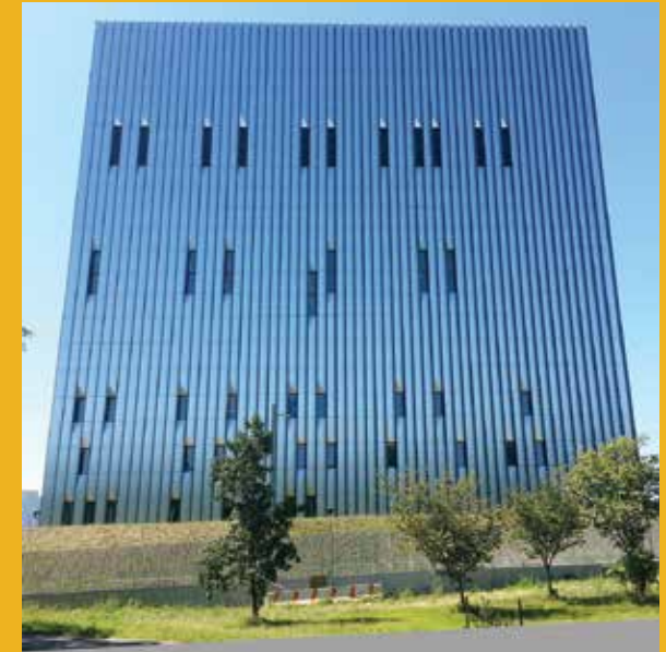
The area of glass on a façade is the strongest predictor of threat to birds. There are also other reasons to limit glass. Skidmore Owings Merrill’s Bronx, New York, Emergency Call Center is a handsome example of creative design with restricted glass, for a building intended to be both secure and blast-resistant. Photo by Chris Sheppard, ABC
