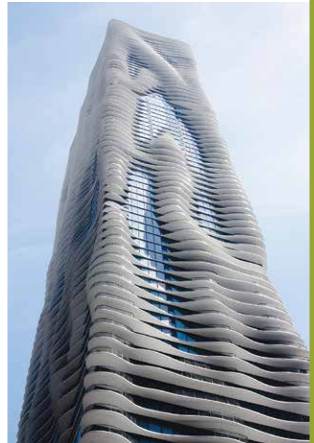
The Studio Gang's Aqua Tower in Chicago was designed with birds in mind. Strategies included fritted glass and balcony balustrades. Photo by Tim Bloomquist
