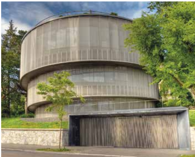
The steel mesh enveloping Zurich's Cocoon in Switzerland, designed by Camenzind Evolution, Ltd, provides privacy, reduces heating and cooling costs, and protects birds, but still permits occupants to see out. Photo by Anton Volgger
