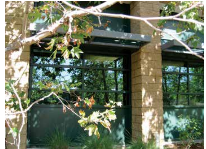
Lower-floor windows are thought to be more dangerous to birds because they are more likely to reflect vegetation. Photo by Christine Sheppard, ABC
