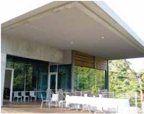
Overhangs block viewing of glass from some angles, but do not necessarily eliminate reflections. Photo by Christine Sheppard, ABC
