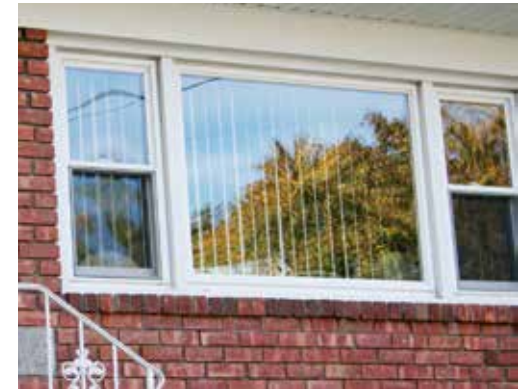
Reflections on home windows are a significant source of bird mortality. The partially opened vertical blinds here may break up the reflection enough to reduce the hazard to birds. Photo by Christine Sheppard, ABC
