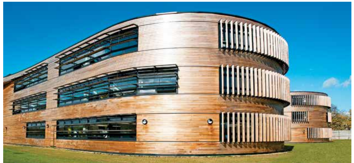
For the Langley Academy in Berkshire, U.K., Foster + Partners used louvers to control light and ventilation, also making the building safe for birds. Photo by Chris Phippen Ofis
