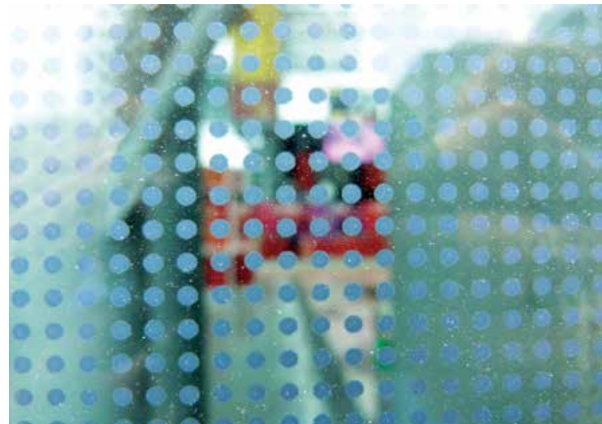
At close range, a visible pattern of frit dots breaks up reflections, making the glass safe for birds. Photos by Glenn Phillips
