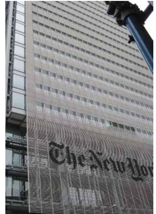
The façade of the New York Times building, by FXFOWLE and Renzo Piano, is composed of ceramic rods, spaced to let occupants see out while minimizing the extent of exposed glass—good for controlling heat and light, and safe for birds. Photo by Christine Sheppard, ABC
